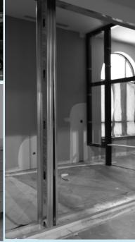
New cabinetry is being installed along the North wall of the sacristy where the sinks were. Much of the drywall has been taped and sanded; the windows frames along Armitage Avenue await stained glass; the reredos panels, a decorative screen behind the altar, have arrived; dark wood paneling is being installed; to the right is a niche for an icon.
