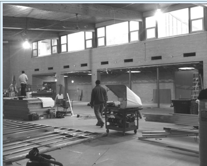
The Terrazzo has now been covered so workers can walk on the floor without damaging it. As of December 17 workers continued with mechanical and electrical construction.
